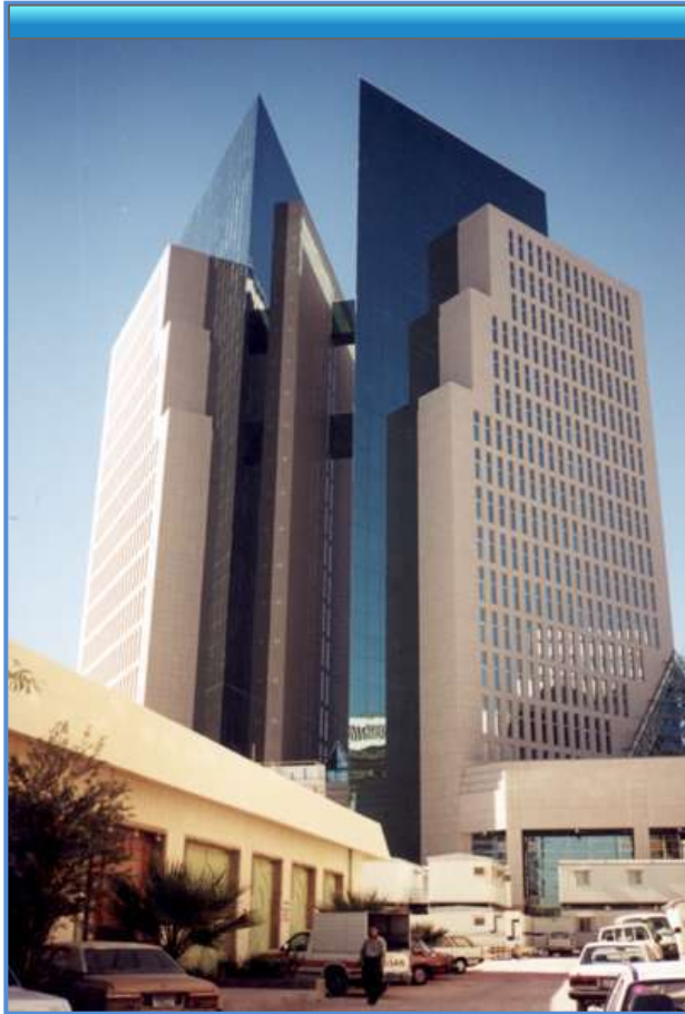
NCCI Tower - Riyadh (KSA) (32 MWh) – (10) TSC-761M
