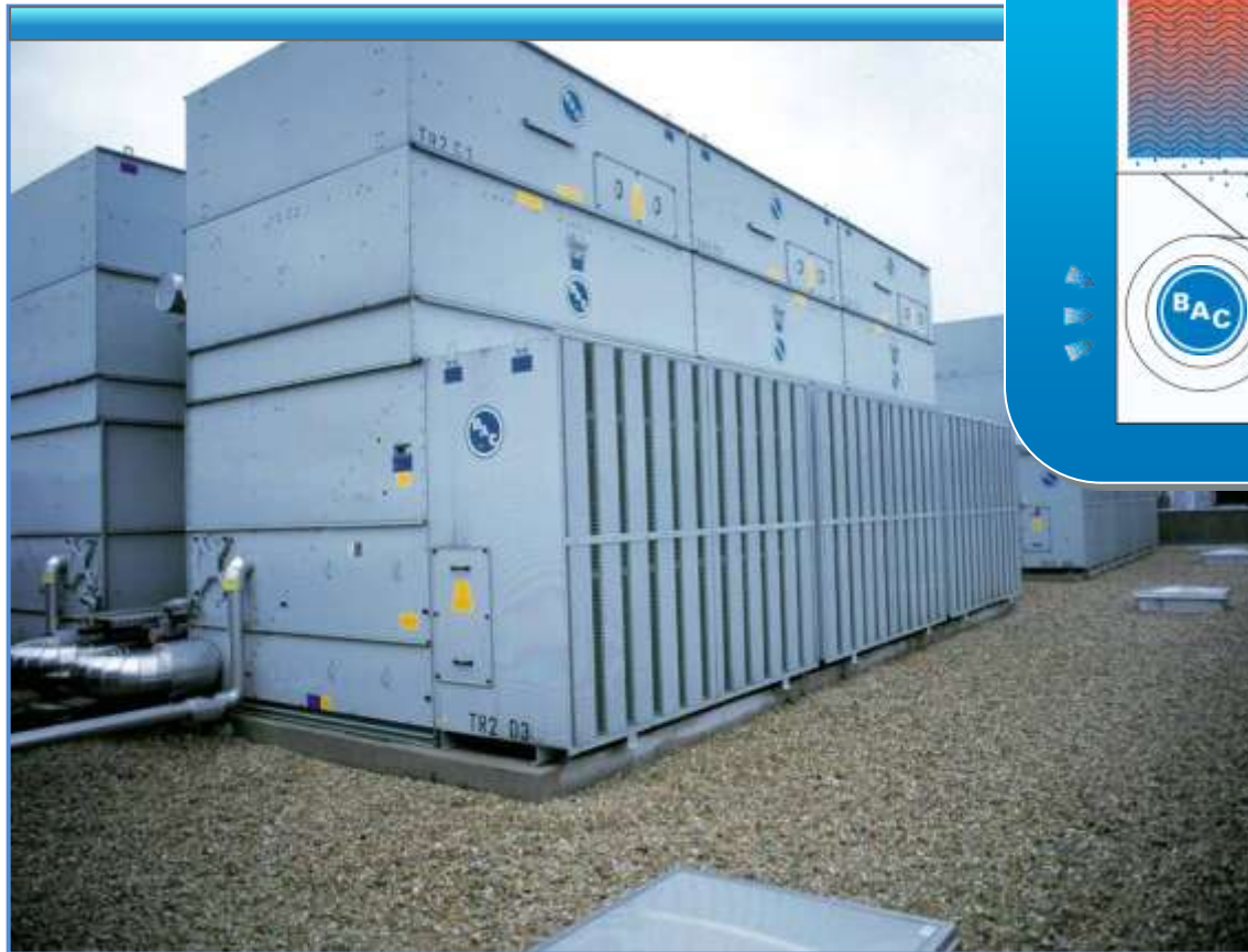
CENTRALE THERMOFRIGORIFIQUE ZAC LANDY Paris, France (4) VXT-945 & (1) VXT-560 20 MW
