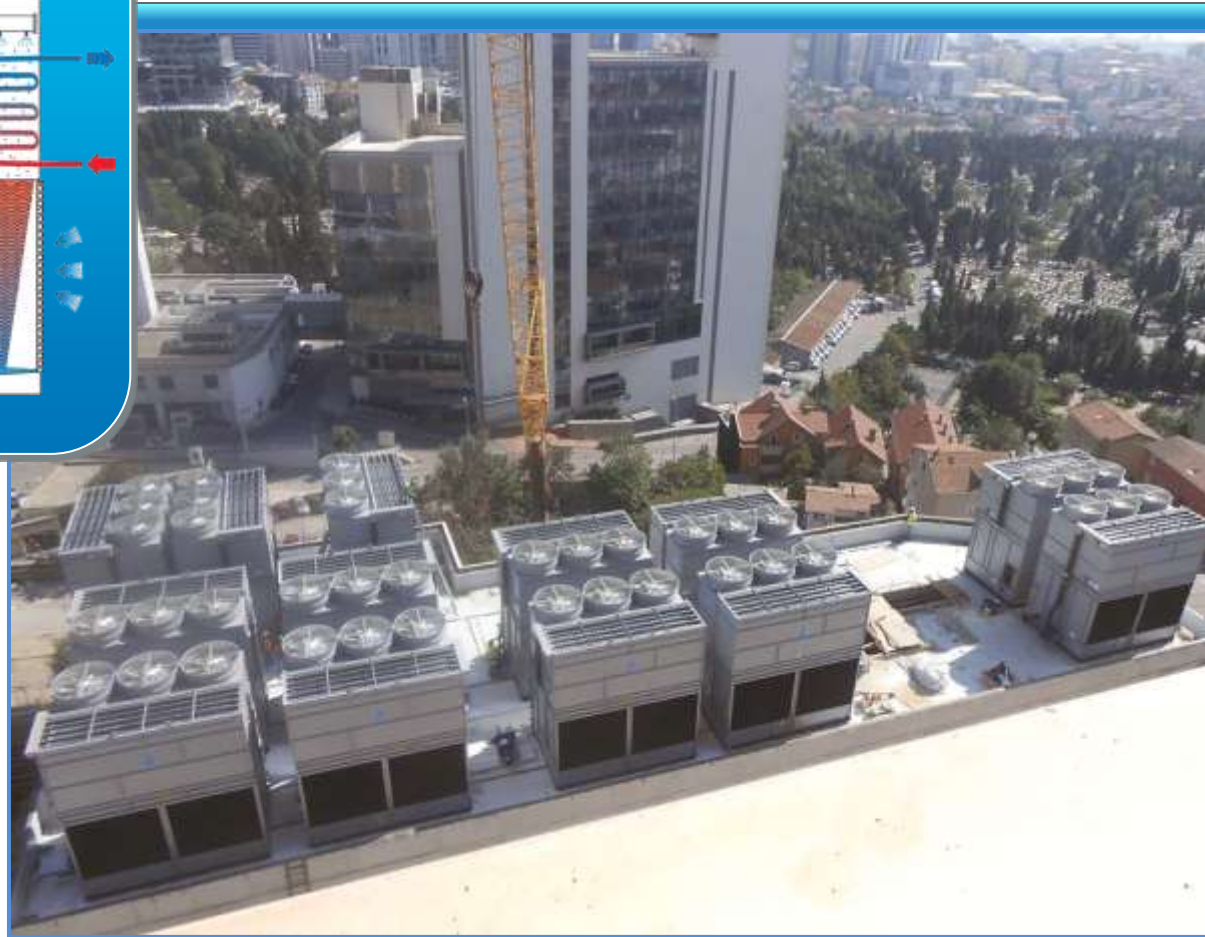
ÖZDİLEK Complex Istanbul, Turkey (13) FXVE units
